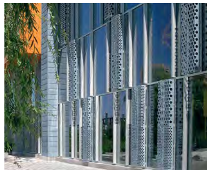
Budynek Boston Children's Museum, Boston, USA
